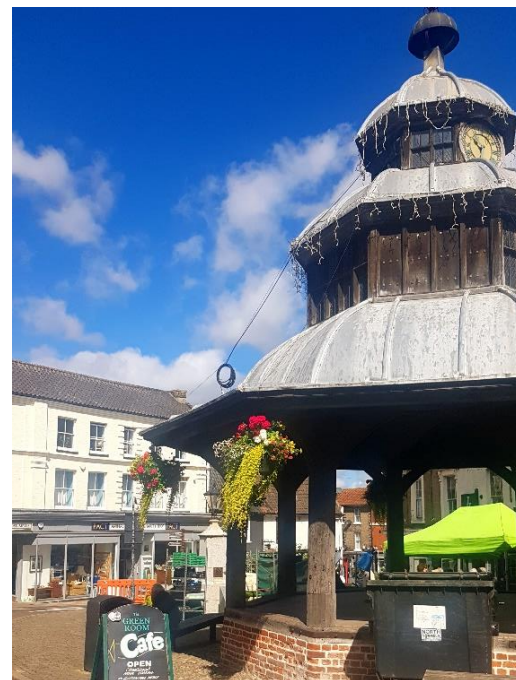
North Walsham Clock Tower
