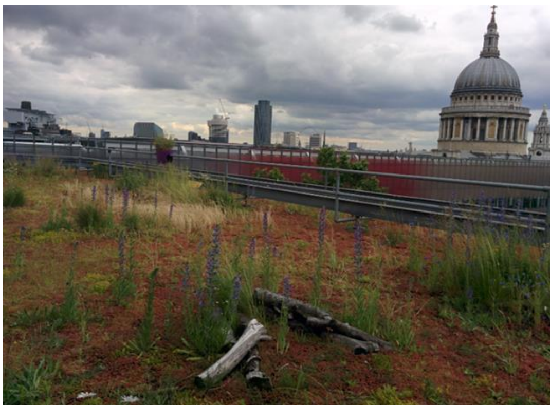
Photo of a green roof with insect habitat, London (Image E Simpson@ NCC LLFA)
