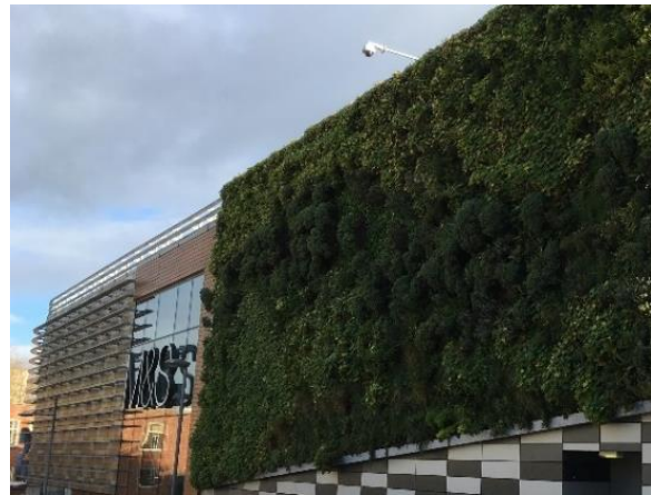
Photo of a green wall on a commercial building in an inner-city area, Norwich, Norfolk (Image E Simpson @ NCC LLFA)
