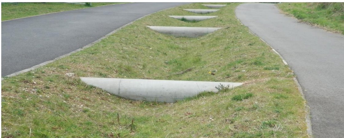
Photo of a swale draining the highway (bus lane and shared use path) located at Queens Hill development, Costessey, Norfolk (image E Simpson @ NCC LLFA)
