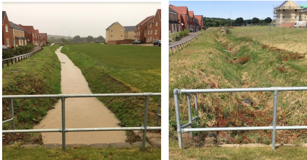
Photos of an ordinary watercourse in North Norwich which is near bank-full during a rainfall event (left) and entirely dry during summer drought (right) (images E Simpson @ NCC LLFA).
