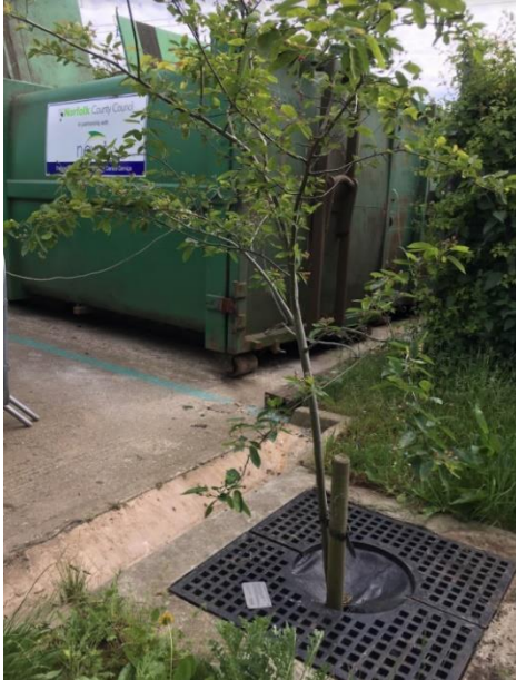
Photo showing example of retrofit SuDS: Tree pit Wymondham NCC Recycling Centre, Norfolk. Treating Surface runoff from the hard standing before discharging to a watercourse.
