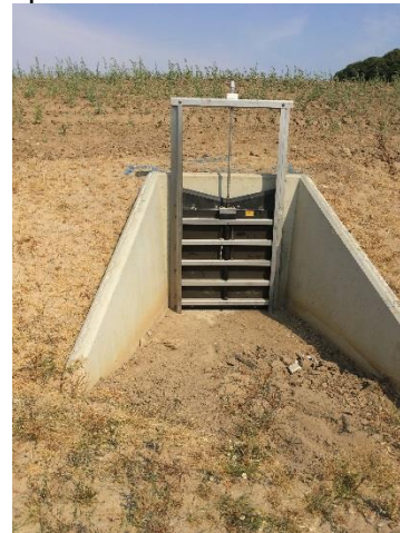
c) Pollution prevention forebay (lined) and outlet to attenuation basin with penstock
