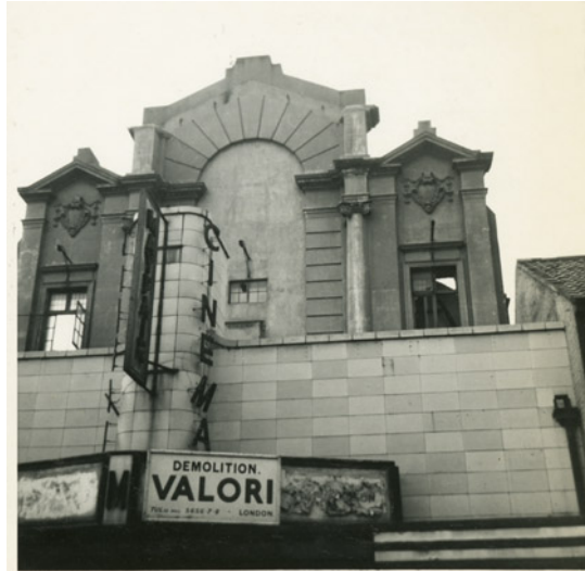
Demolition of the Mayfair Cinema, Magdalen Street Norwich, 1962
