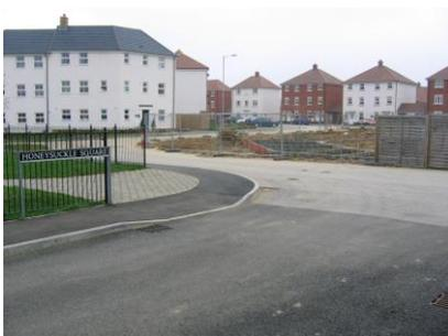
Whilst development is being built, units will inevitably be occupied. Therefore the roads/footways need to be constructed to a suitable temporary standard to be used by residents which is normally the course below the surface course (binder course). The surface course is not laid until construction has finished but must be laid prior to Condition *SHC 02* being discharged.
