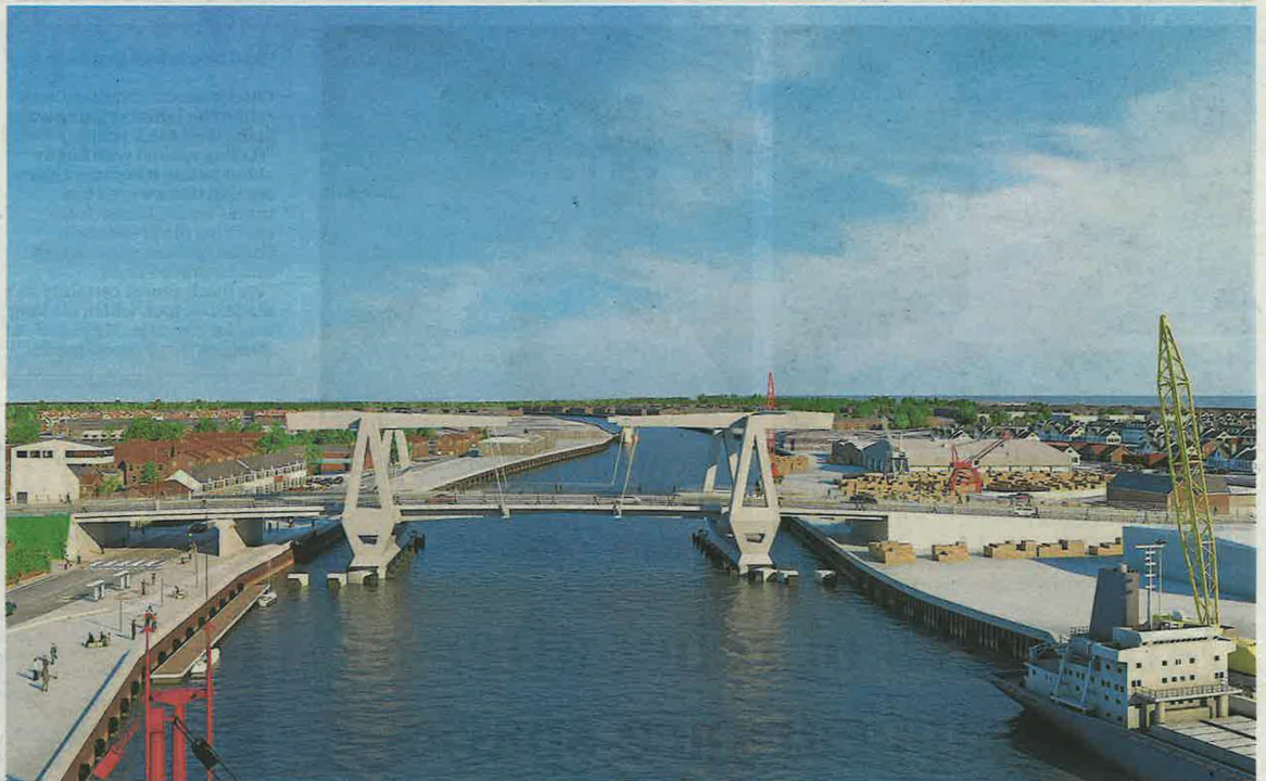
Illustrative design to show one of the opening mechanisms being considered for the third river crossing in Great Yarmouth
