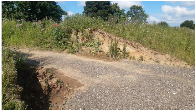
11. Parcel 7 - southern verge and bund (June 2021)
