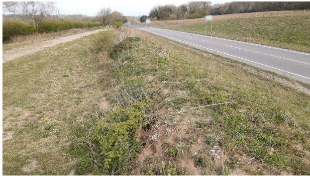
9. Parcel 7 - southern verge and bund in foreground, northern verge to right of picture (April 2021)
