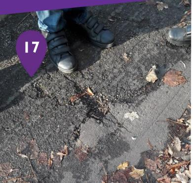
The surface is very rough with tarmac eroded out and cracks 3-4cm across
