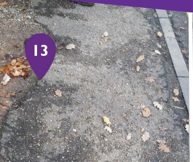
The path has become eroded at one side which has created a cross gradient of 1:11. There are small drainage gutters creating a 10mm dip across the path at intervals for 15m
