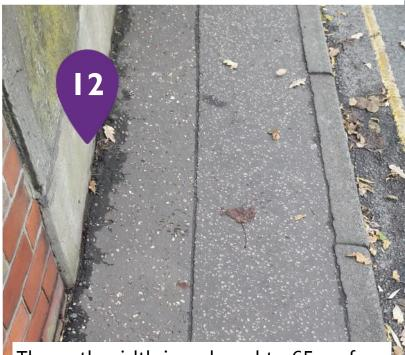
The path width is reduced to 65cm for 20m. There is also a cross gradient of 1:11 where the dropped curbs at each crossing has cut into the footpath
