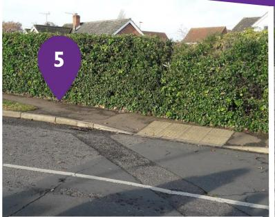
There is a gradient of 1:6.2 at the dropped kerb at the crossing over Skeyton New Road. There are cracks 5mm across in the tarmac in the road which has created an uneven surface
