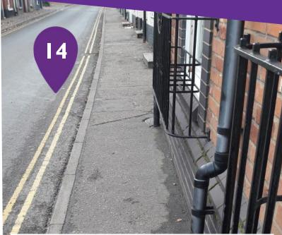
The path width is reduced to 50-55cm at intervals for 100m due to several window box grates and door steps cutting into the footpath
