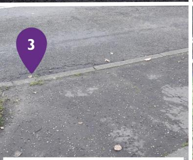
There is a dropped kerb on both sides of Station Road with a 10mm step. There are cracks in the tarmac on the road ranging from 5mm to 10mm creating a slightly uneven surface
