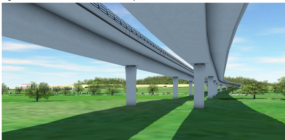
Figure 17: Soffit of Concrete Box Girder Option.
