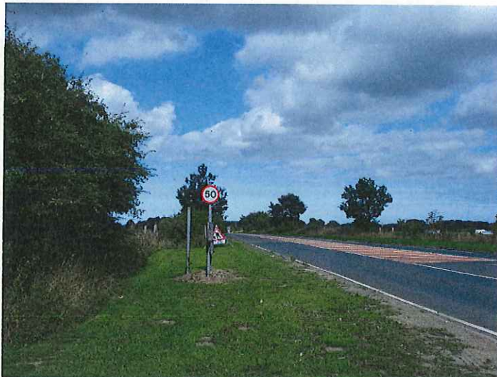
Bushes (behind sign array) obstructing visibility splay
