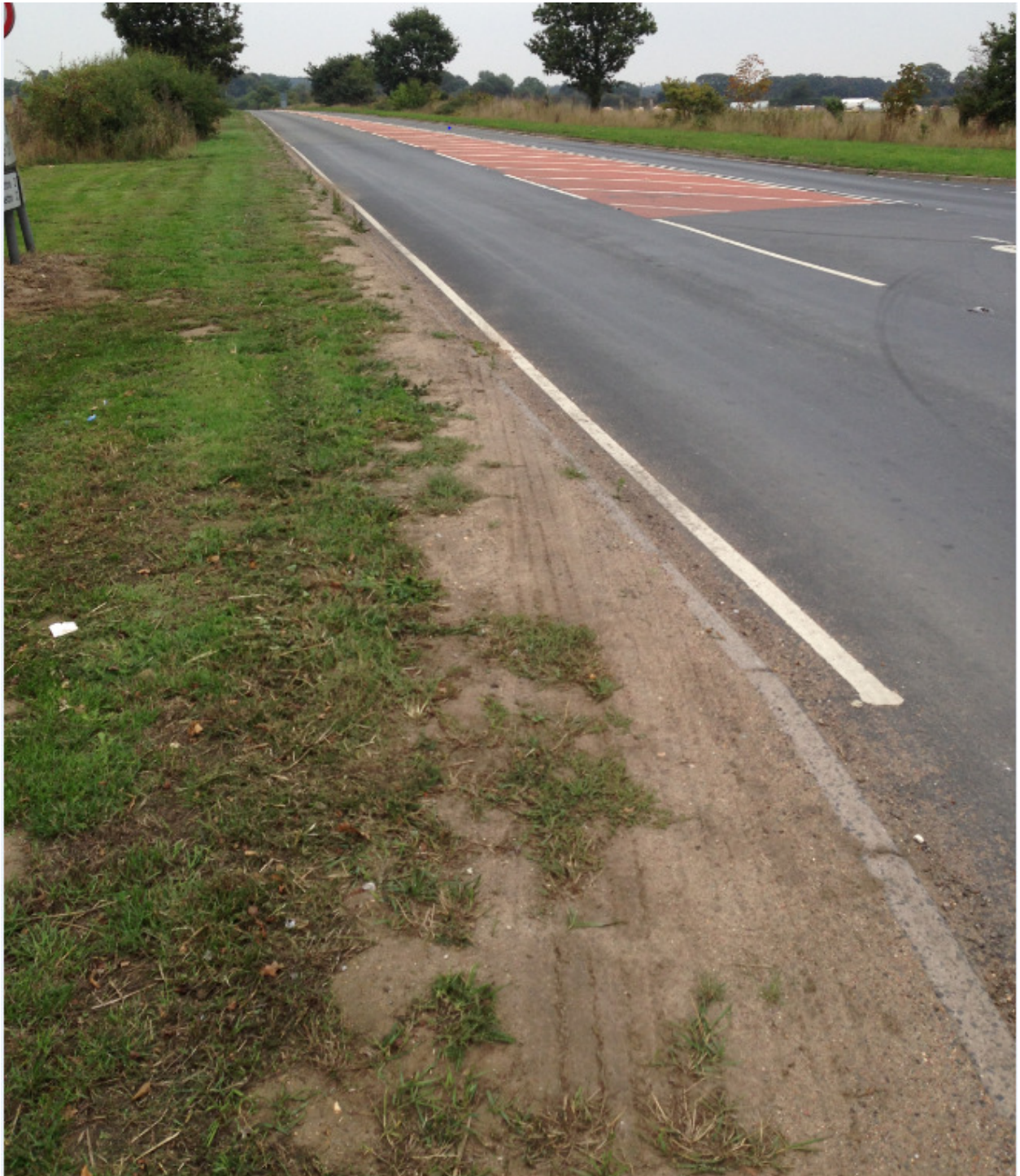
PHOTO 3 Facing Northeast at the bell mouth of Crostwick Lane
