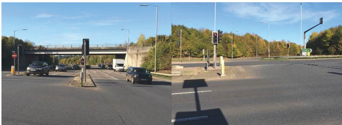
Photo 5.1 Existing Junction Layout – A47(T) / A146 South-Eastern Junction
