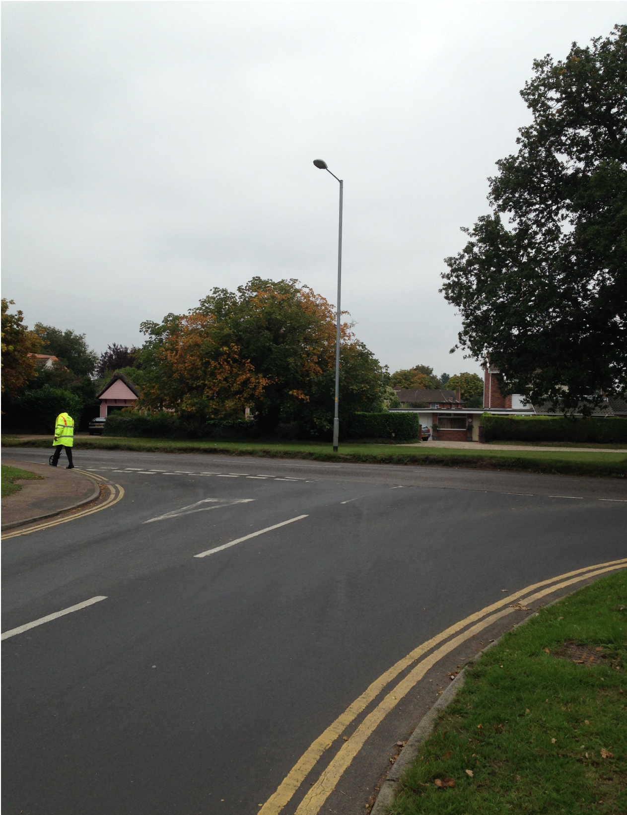
PHOTO 1 Facing East on Broadland Drive
