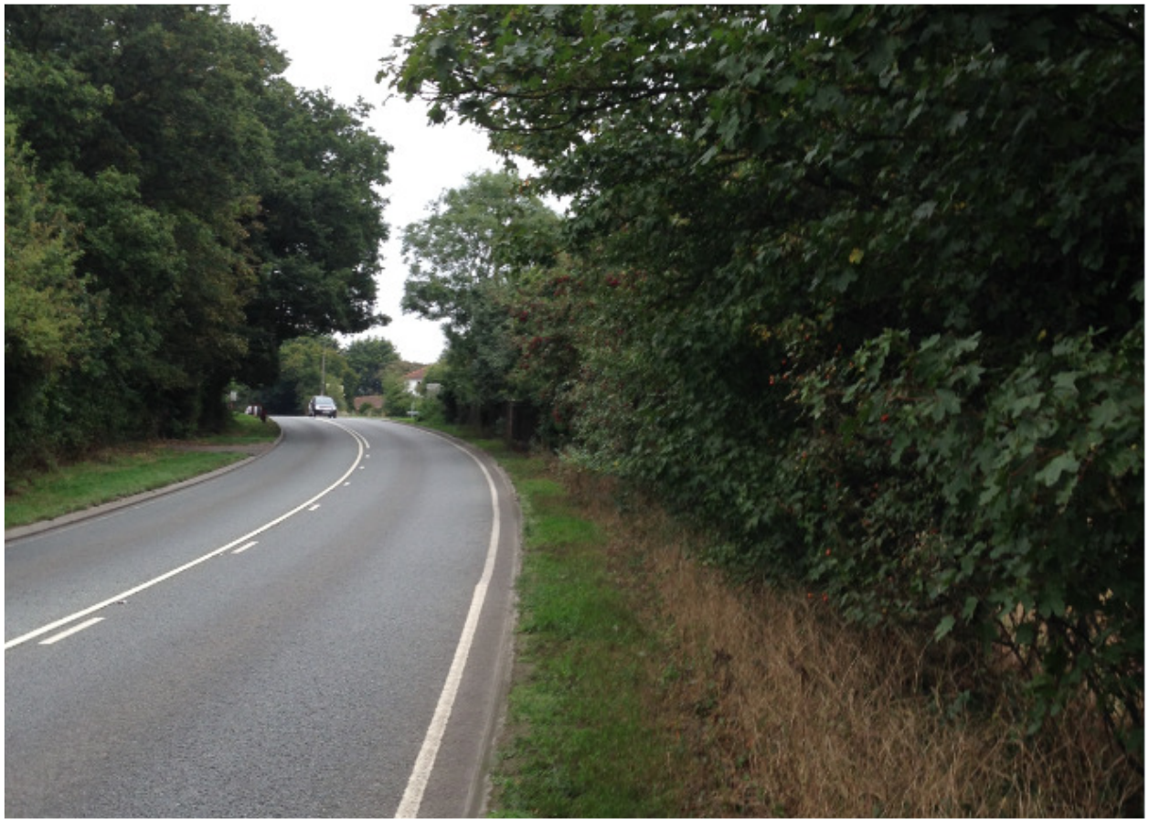
PHOTO 7 Facing Northeast at the right side kerb of Wroxham Road (A1151)
