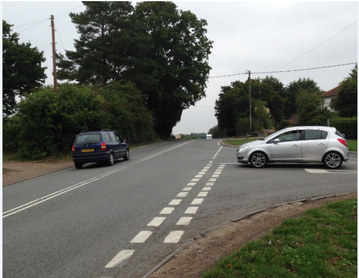
PHOTO 5 Facing Northeast at the right side kerb of Wroxham Road (A1151)
