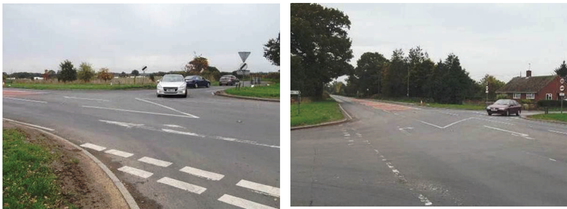
Photo 5.4 Existing Junction Layout – North Walsham Road / Rackheath Lane
