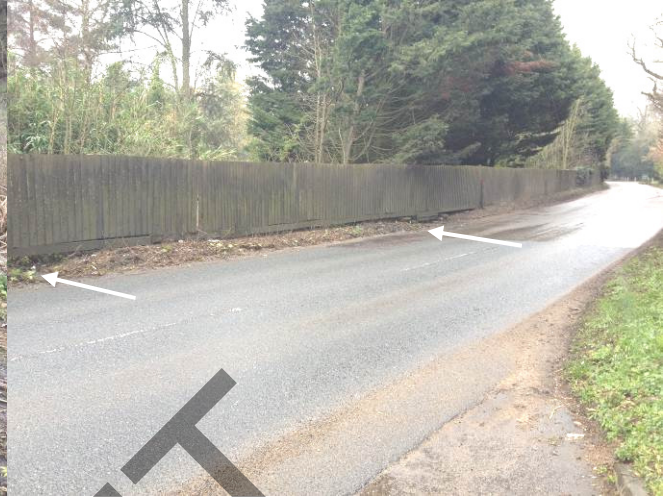
Photo 3.2: Grips under fence (white arrows) between Weston Hall and A1067, draining to a ditch which flows to the Wensum.
