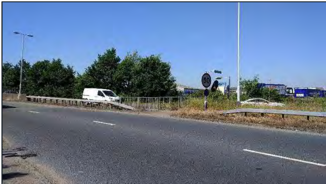
Informal pedestrian crossing facilities across the A47
