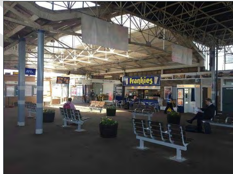
Great Yarmouth Main Station Building
