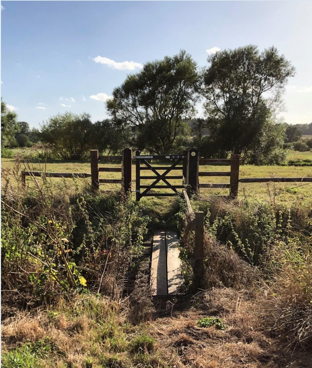
Figure 2-33 - Site 7, Narrow bridge across watercourse
