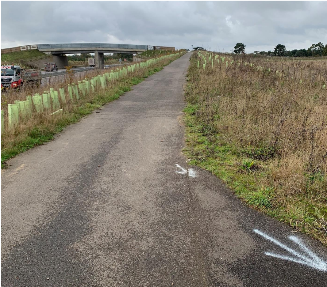
Figure 2-53 – Marriott's Way bridge, access from Furze Lane
