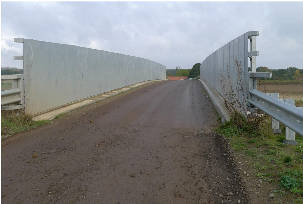
Figure 2-52 - Horsford RB5 bridge parapet
