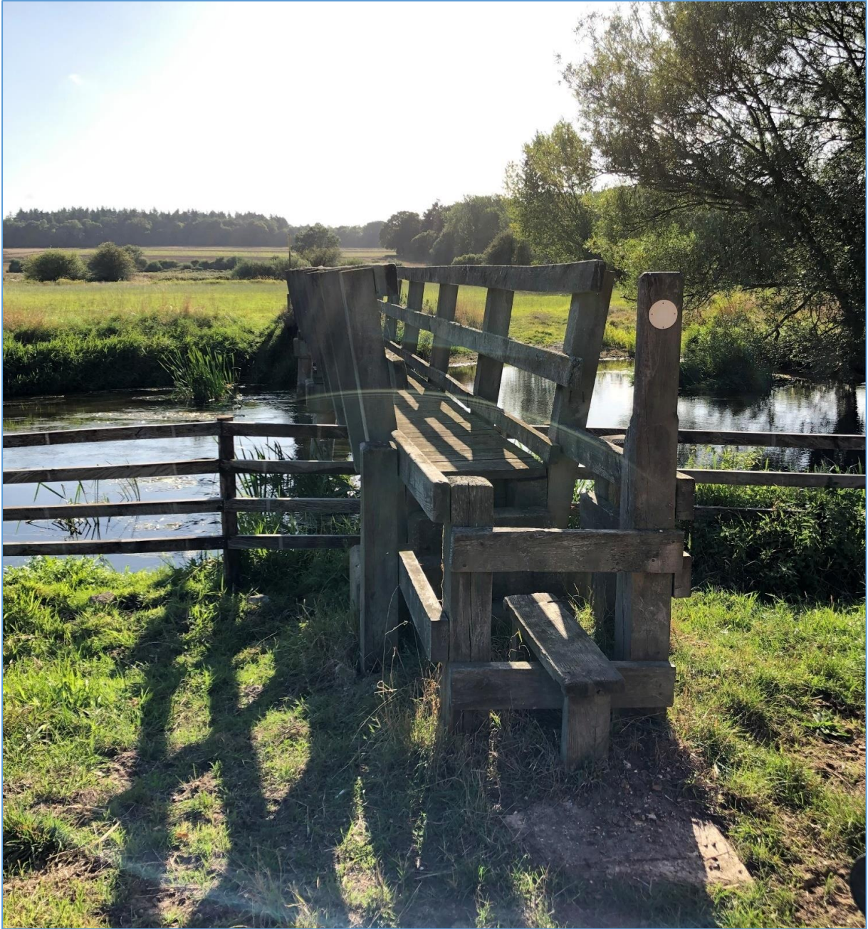
Figure 2-35 - Site 7, Footbridge across the River Wensum
