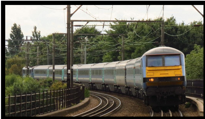
Picture: Two-track section of Great Eastern Mainline at Chelmsford
