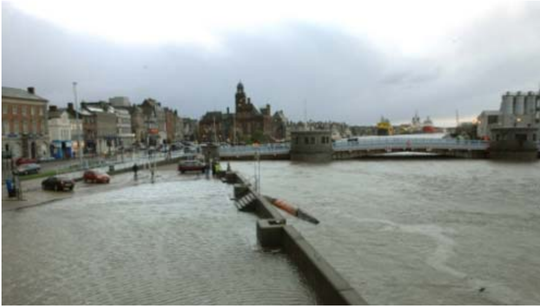
Figure 2-27 Flooding in the vicinity of Haven Bridge
