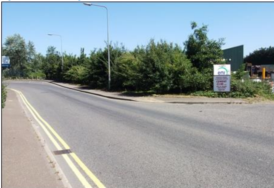
Figure 3.1: Ernest Gage Avenue and the access to EMR and Norfolk Cement
