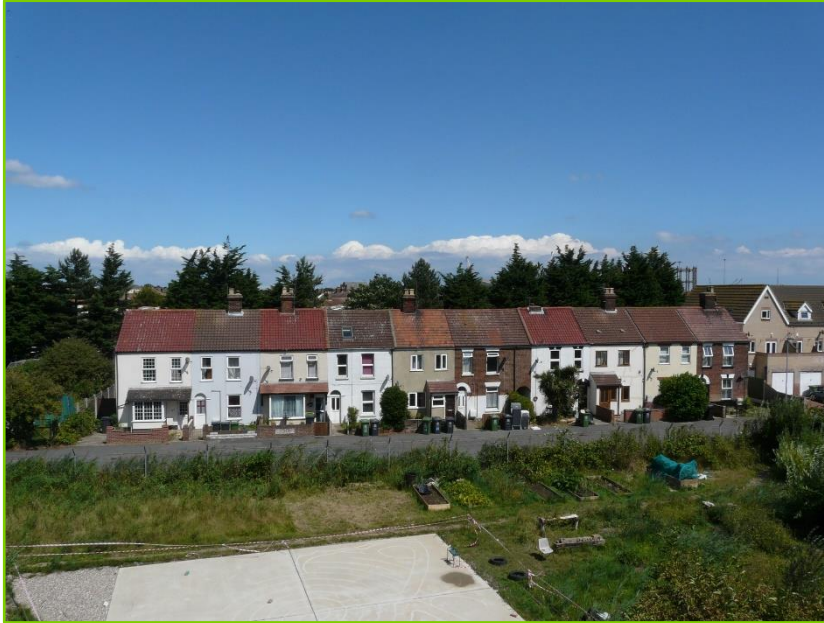
Plate 9.2: WSP04: Late 19 th Century Terraced Housing on Queen Anne's Road
