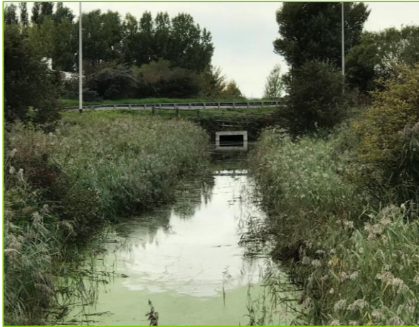
Plate 11.6: On Pasteur Road looking downstream (west) towards the A47 Culvert
