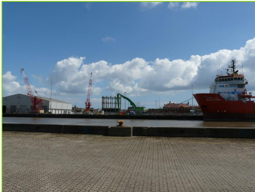
Plate 9.10: View East Towards the Gas Holder (NHLE 1096789) from Southtown Road
