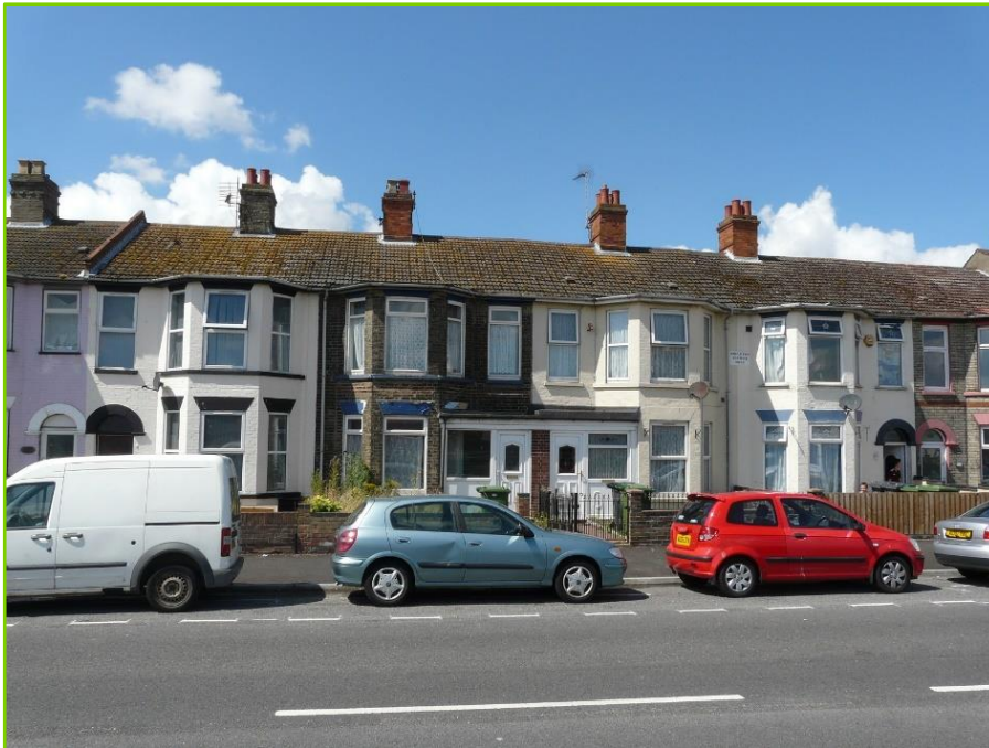
Plate 9.1: WSP06: Late 19 th Century Terraced Housing on Southtown Road
