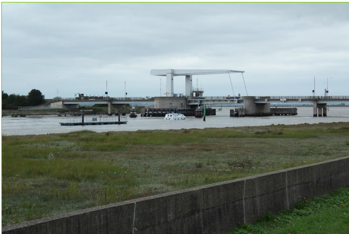
Plate 10.8: View of Breydon Bridge from Path adjacent to Asda Supermarket
