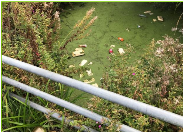
Plate 11.8: The drain that runs from south to north, downstream of the William Adams Way culvert
