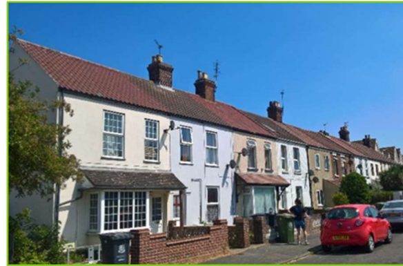
Plate 12 – Buildings B1, assessed for bat roost potential
