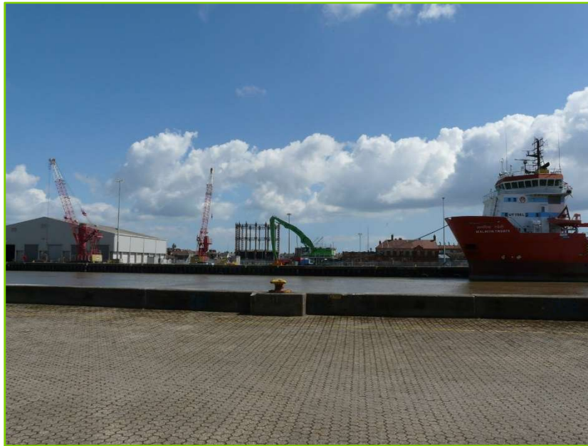
Plate 7.11: View East towards the Gas Holder (NHLE 1096789) from Southtown Road
