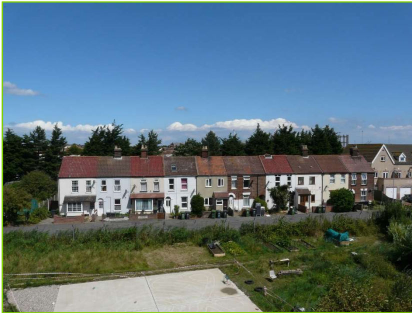
Plate 7.2: WSP04: Late 19 th Century Terraced Housing on Queen Anne's Road
