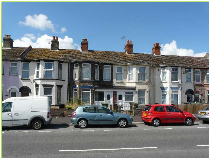
Plate 7.1: WSP06: Late 19 th Century Terraced Housing on Southtown Road
