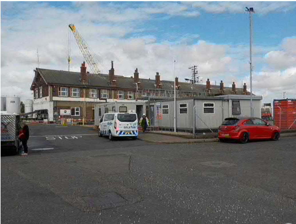
Photograph 8 – Access to Butler Fuels and quayside properties from South Denes Road
