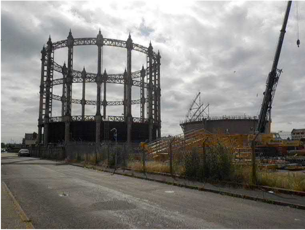
Photograph 1 – Barrack Road Gasworks
