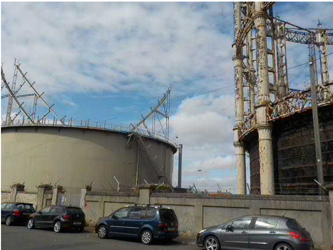
Photograph 2 – Barrack Road Gasworks
