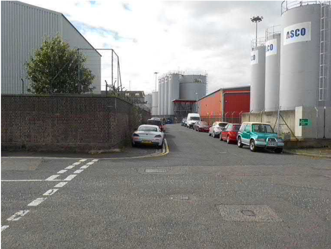
Photograph 5 – ASCO Ltd storage tanks
