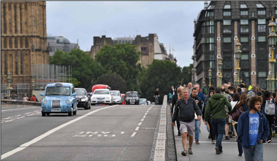
Plate 1 - Varioguard type barriers between cycle/bus lane and footway on Westminster Bridge
