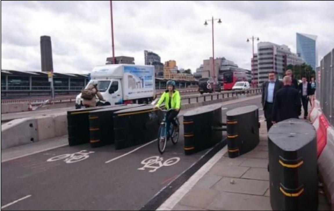
Plate 4 - VSBs providing a gap of 1.2m to allow cycle and pedestrian access on Blackfriars Bridge. Again, the size of these units is dictated by the lack of foundation available on the bridge deck, which would, if available, allow much smaller bollards to be used.
