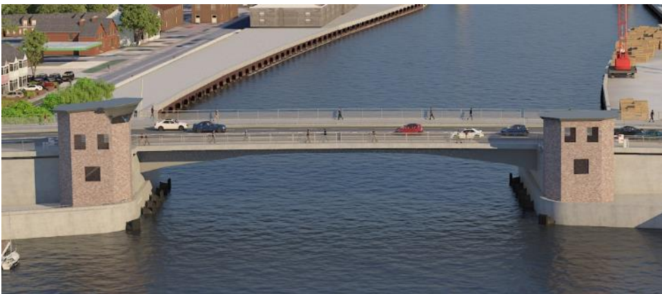
Figure 6-11: Indicative render of how the Control Tower and Plant Room structures could look
