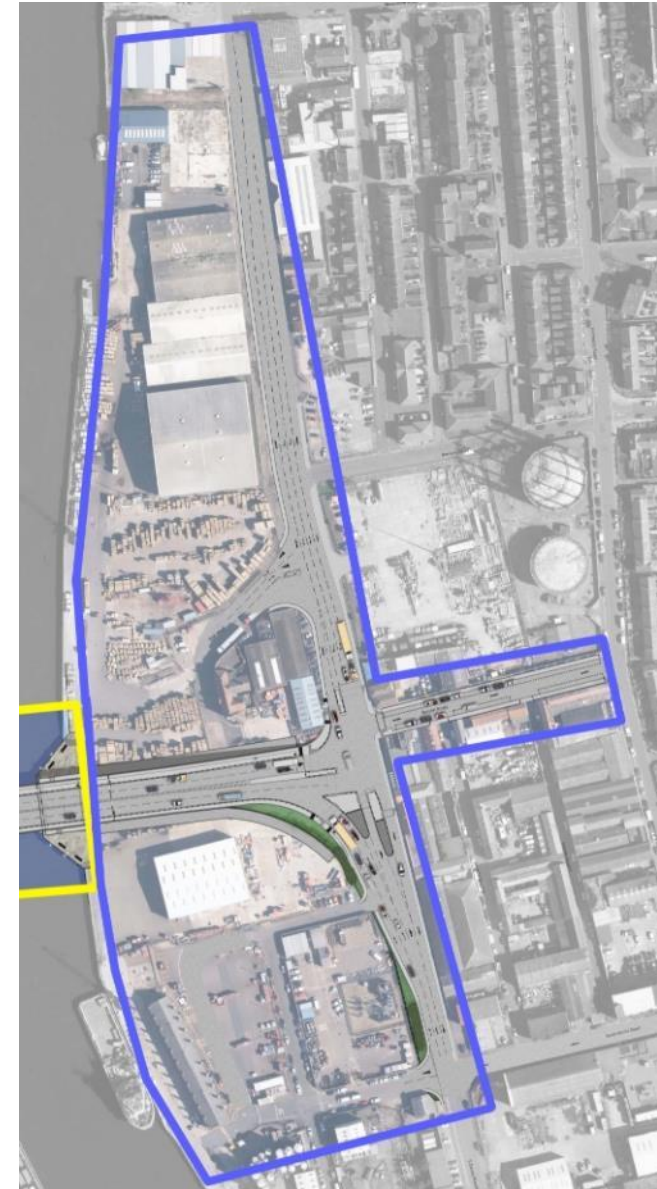
Figure 6-14: Eastern approach area of the Scheme
