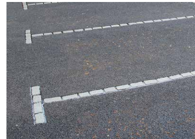
Coloured chipped macadam and block pavers for bay demarcation
