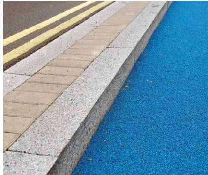
Cycle track and kerb
