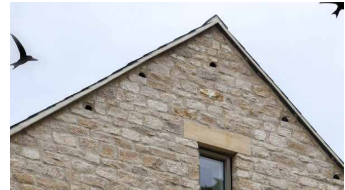
Example of bird boxes in a structure
