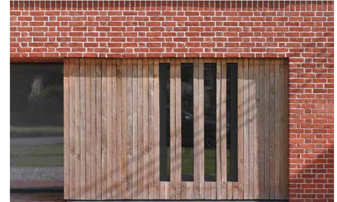
Example of using brick and timber
