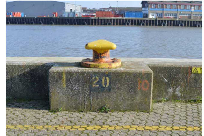
Existing quay wall on Bollard Quay
