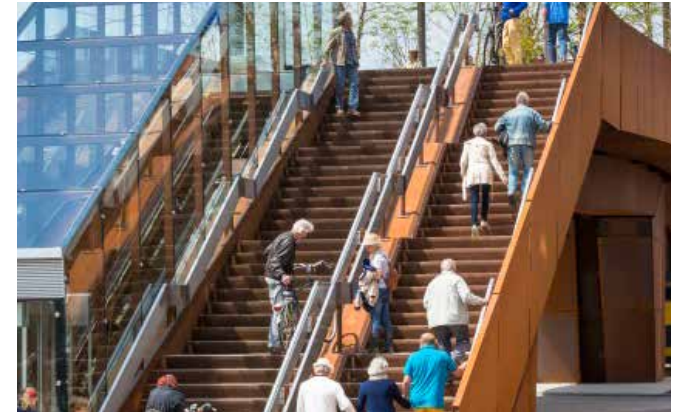
Example of public stairs and a cycle wheeling ramp
