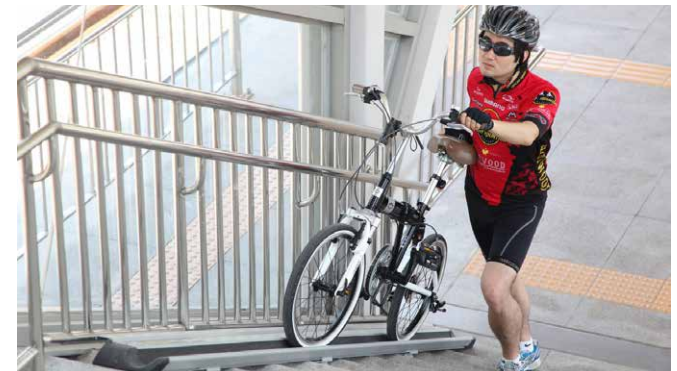
Example of a cycle wheeling ramp
