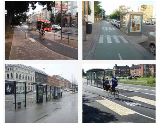
Examples of bus stop bypasses
