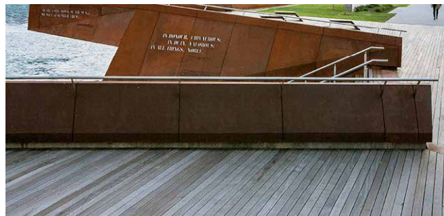
Example of a quay wall and hand rail
