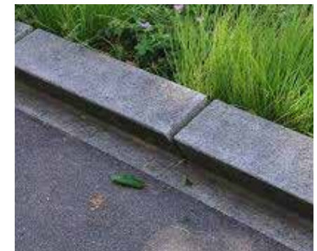
Kerb drains for SuDS
