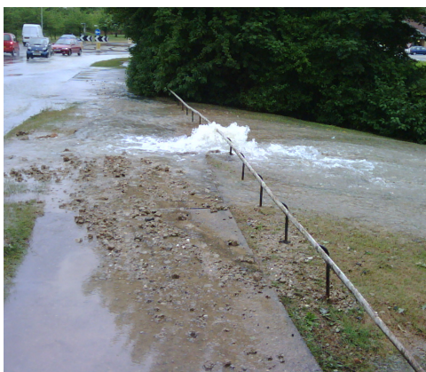
Figure 4-3 Surcharging of the sewer system within a road (left) and internally within a property (right)
