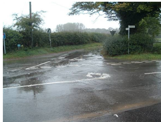
Surcharged sewer on Waters Lane, Hemsby, October 2008
