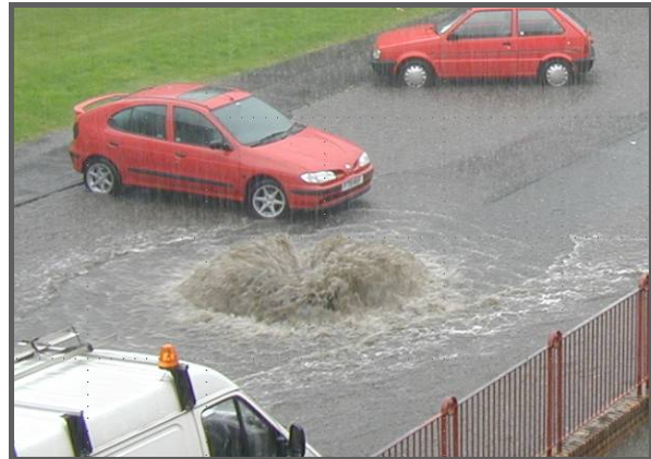
Figure 4-1: Surcharging of the sewer system
