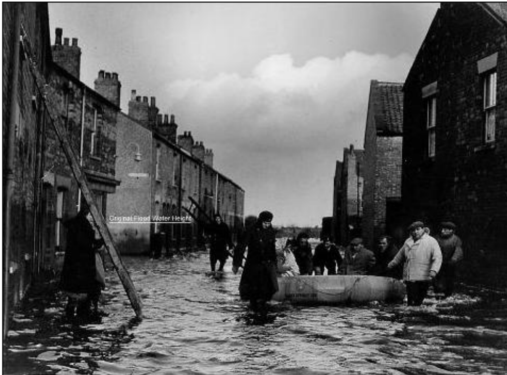
Figure 2-1 Flooding in King's Lynn from the 1953 East Coast Floods 2
