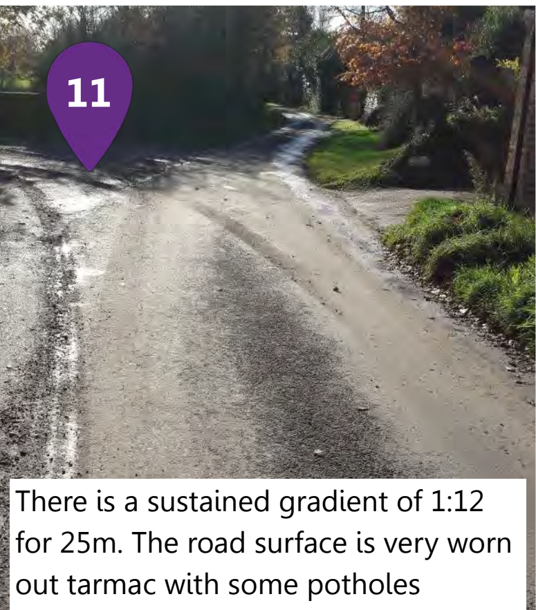
The tarmac on the road surface has become very worn out and there is rutted grass and loose material in the centre
