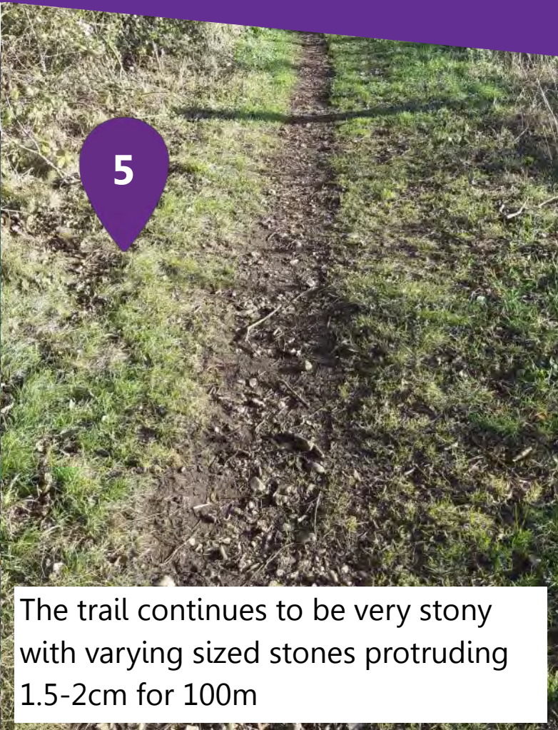
There is a gradient of 1:7 on the approach to Canal Farm Lane crossing. The surface is very stony and uneven with rutted grass. The trail width continues to be narrow at 20-40cm across due to the encroaching vegetation on either side of the trail
