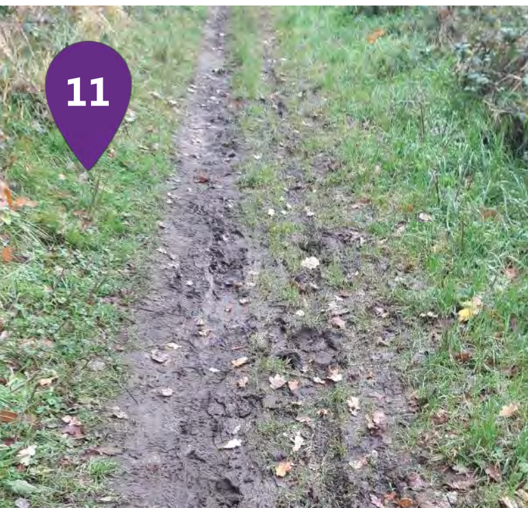
There is a split level path for 25m which reduces the trail width to 35cm
