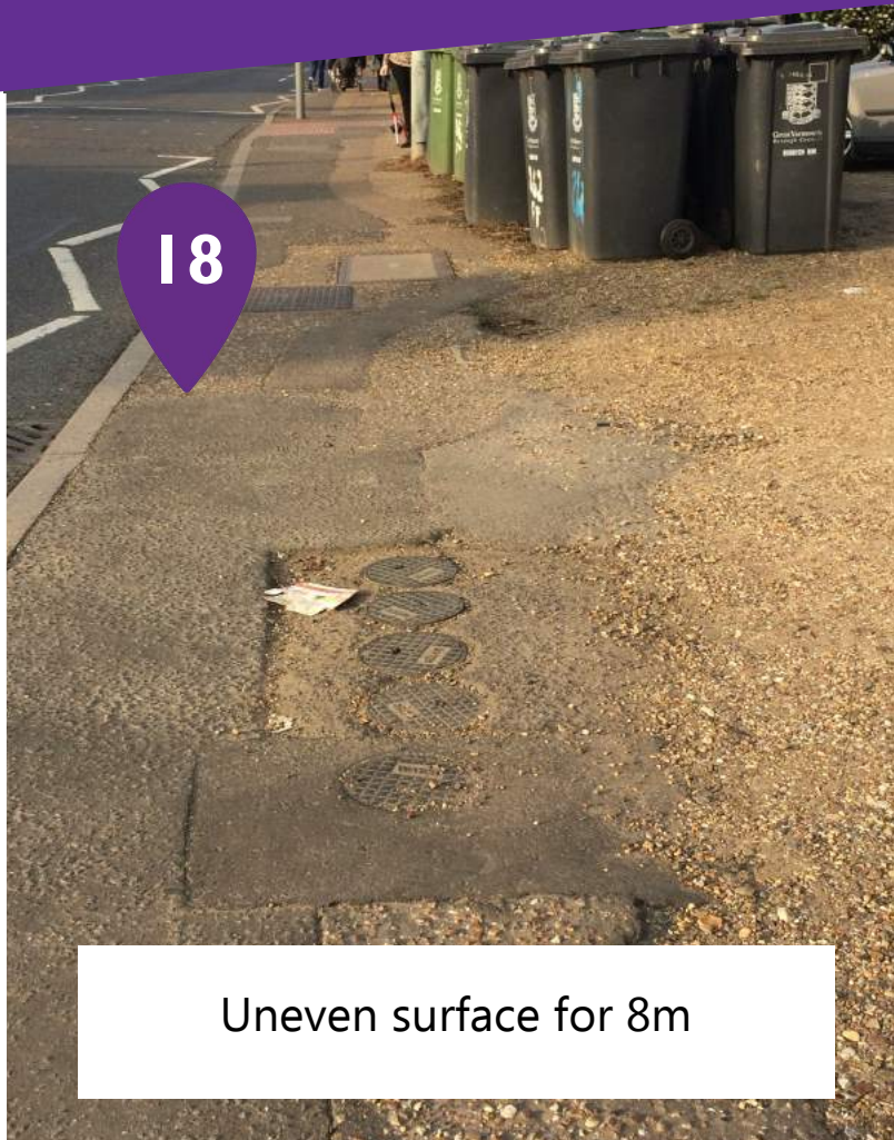
Uneven surface of footway for 6m
