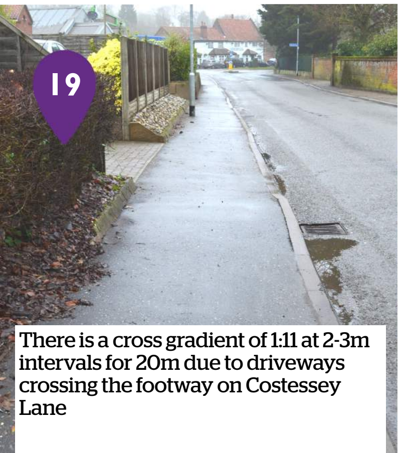
At Costessey Lane, there are no corresponding dropped kerbs to cross the road. Users may need to travel along the road for 4-5m to reach the dropped kerb on the opposite path
