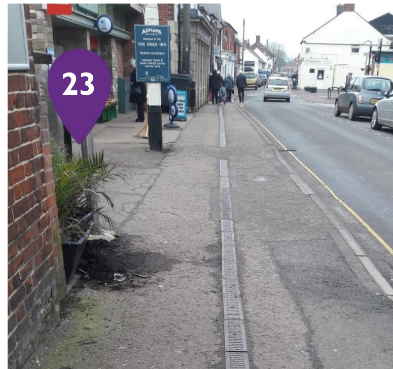
There is a drain grate in the centre of path with gaps between the plates around 1.5cm for 42m
