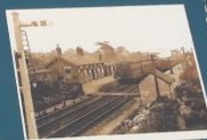
View from the railway bridge looking towards Great Yarmouth
