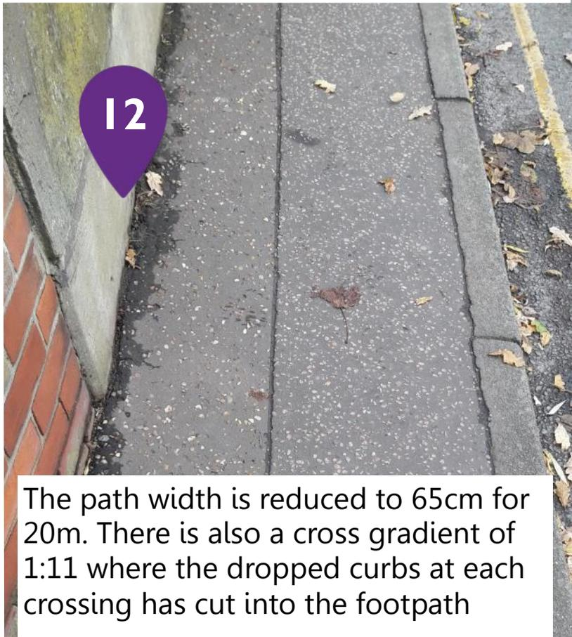
The path width is reduced to 65cm for 20m. There is also a cross gradient of 1:11 where the dropped curbs at each crossing has cut into the footpath
