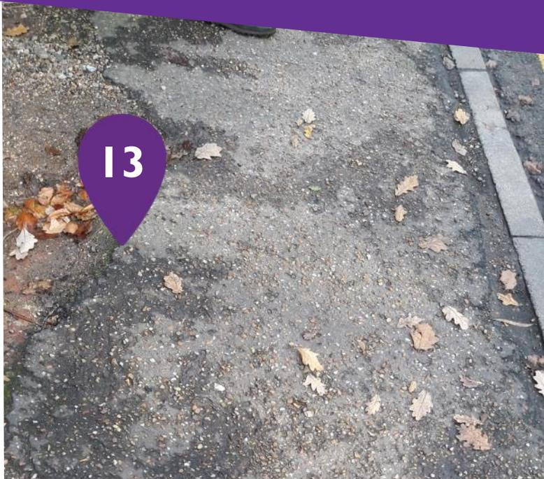
The path has become eroded at one side which has created a cross gradient of 1:11. There are small drainage gutters creating a 10mm dip across the path at intervals for 15m
