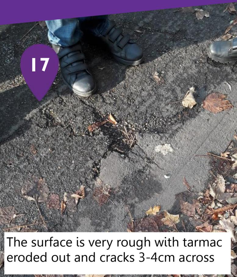
The surface is very rough with tarmac eroded out and cracks 3-4cm across
