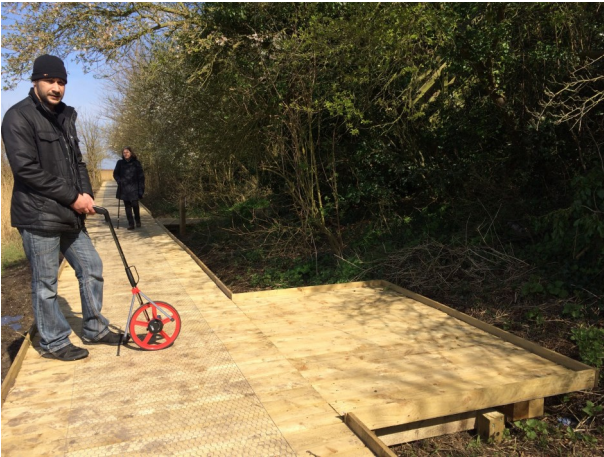
Wide platform area
