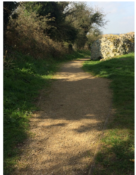
Surface: constructed and firm (compacted limestone), some small loose stones Start of gradient
