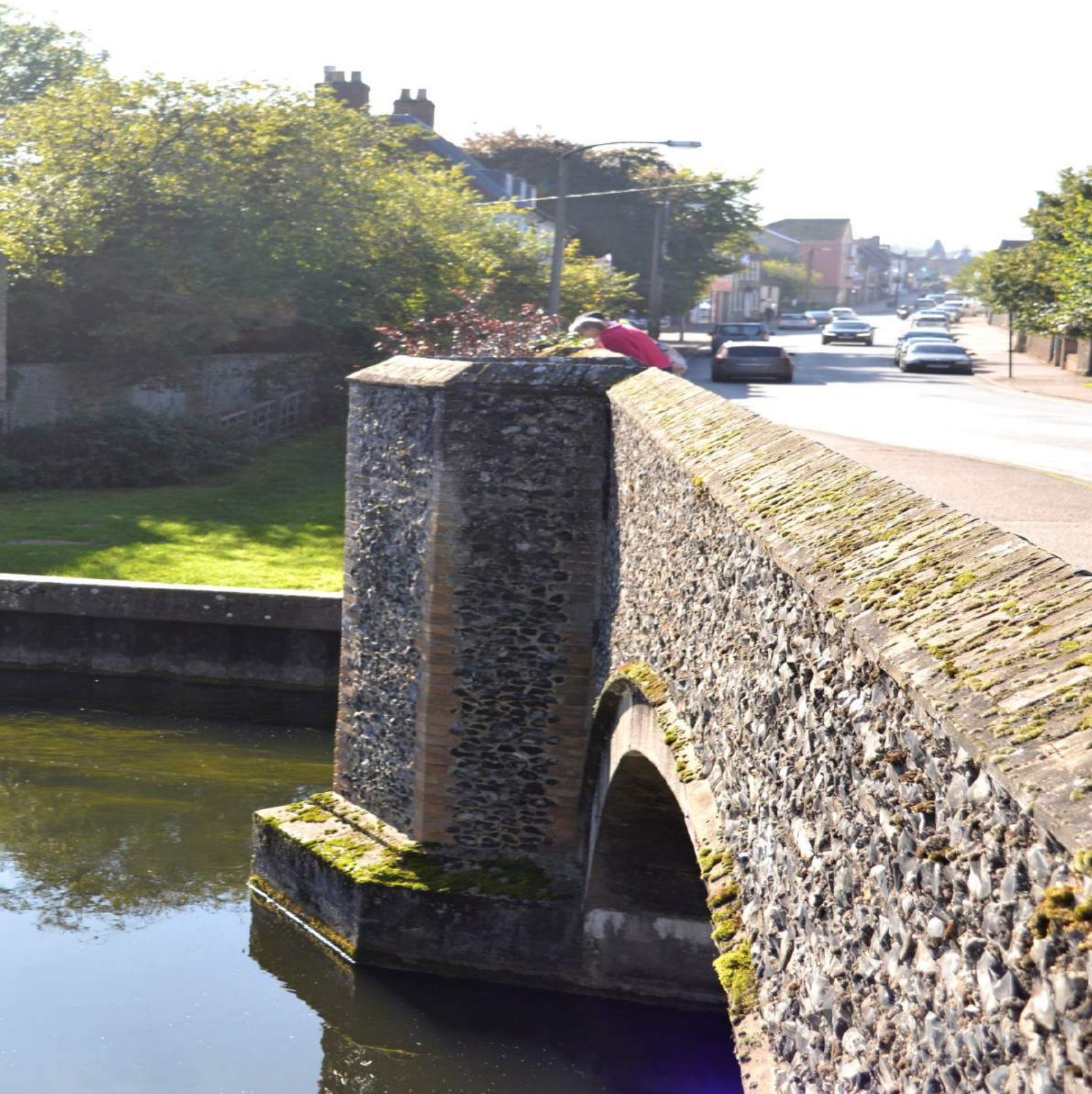
Bridge over the Little Ouse River
