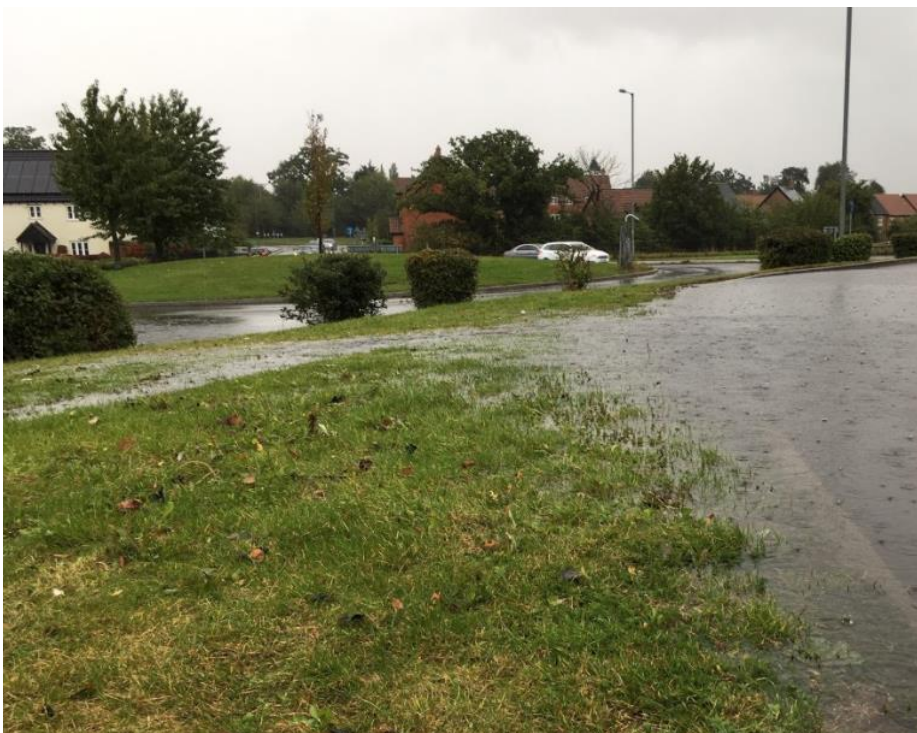
Photo of Surface Water Flooding in North Norwich (Oct 2019): Surface water in a petrol station and car park, overtopping the kerb, leaving the site uncontrolled and flooding the highway. The traditional drainage system was overwhelmed. Flooding also occurred in 2016 causing significant traffic disruption (Image from E Simpson @ NCC LLFA).
