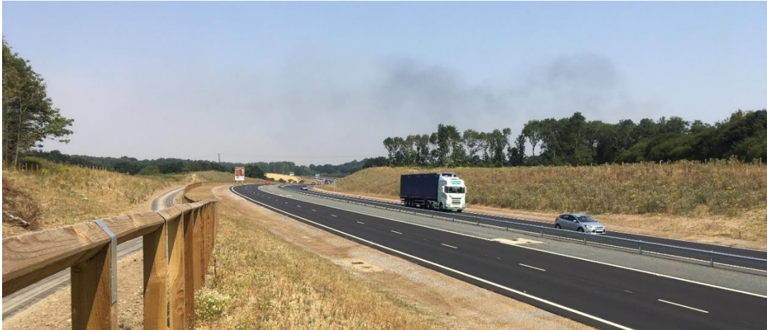
Photo of a newly created swale with over the edge drainage on Broadland Northway, Norwich, Norfolk (Image E Simpson @ NCC LLFA)
