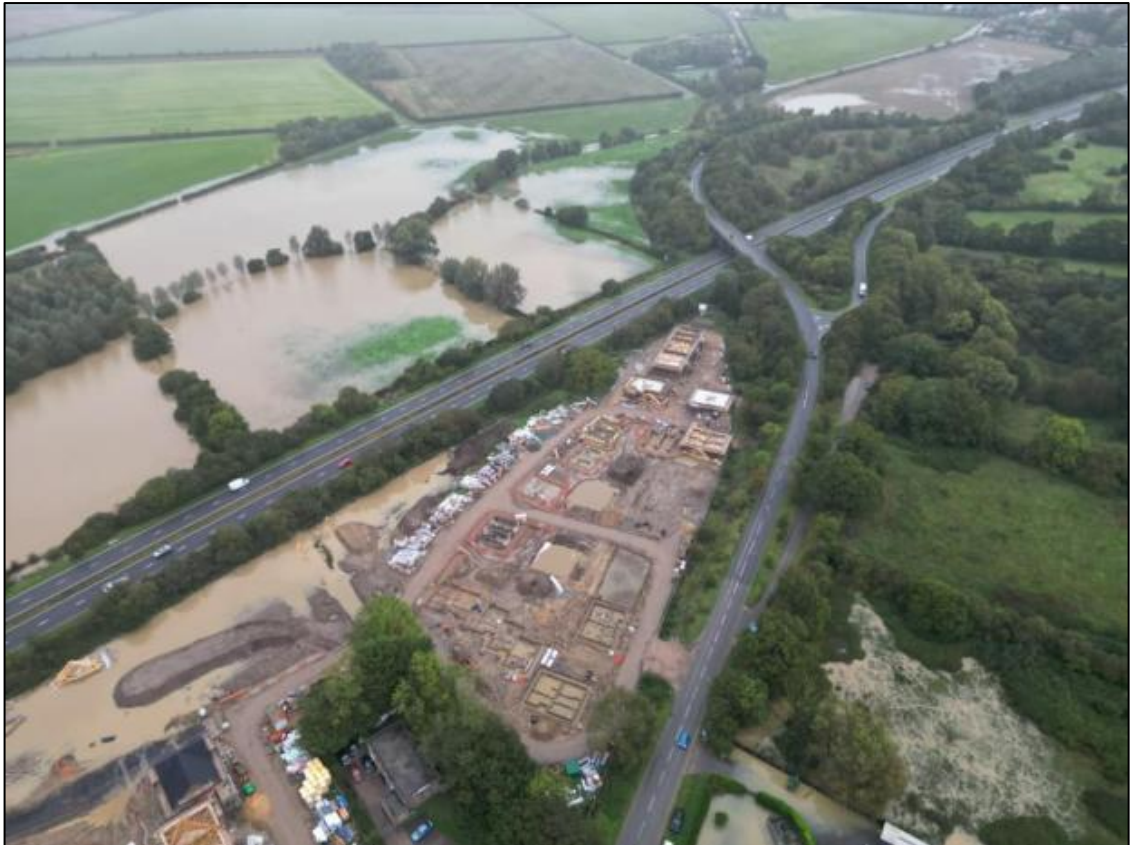
Photo of a development site located on the mapped surface water flood path that flooded in 2023, Attleborough, Norfolk. Source: Wymondham and Attleborough Mercury, October 2023.
