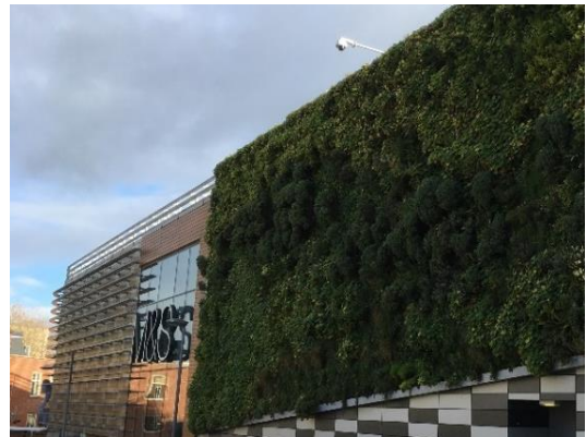
Photo of a green wall on a commercial building in an inner-city area, Norwich, Norfolk (Image E Simpson @ NCC LLFA)
