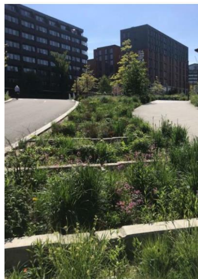
Photo showing example of retrofit SuDS: Planter with under drained raingarden, over edge drainage from the highway and paths. Sheffield Grey to Green Project.
