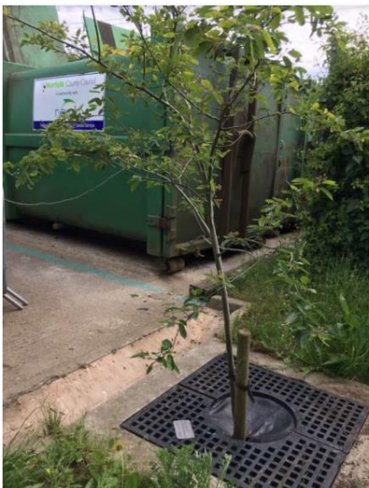
Photo showing example of retrofit SuDS: Tree pit Wymondham NCC Recycling Centre, Norfolk. Treating surface runoff from hard standing before discharging to watercourse.
