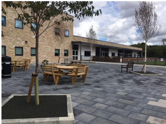
c) Under-drained permeable paving in outdoor dining area
