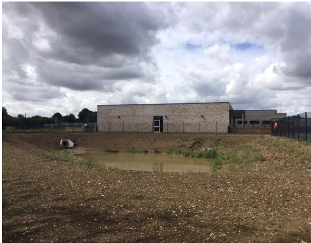
e) Main attenuation basin within two inlets, (silt in basin from jetting of pipe network on day of photograph)
