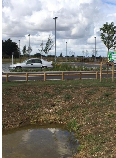
b) Offline attenuation area with low fencing at front door of building
