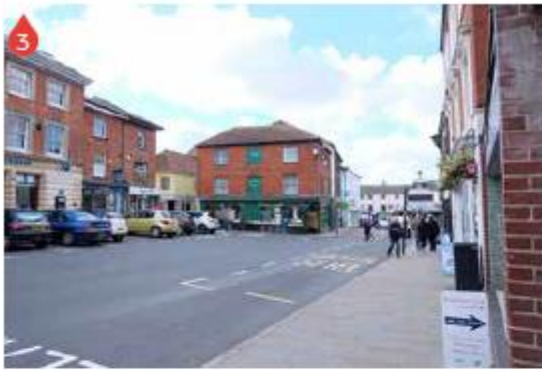
Insufficient footway space at bus stop for alighting and boarding Lack of crossing points Wide carriageway area to cross between the two sides of the street
